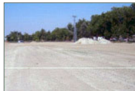
Röske after stabilization
