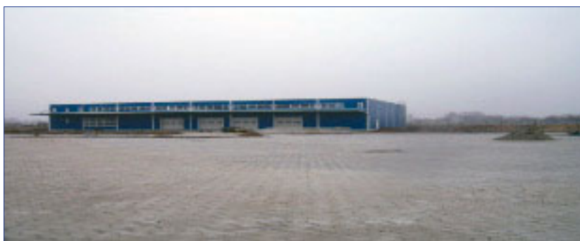
Truck parking and storage facility, Röske, Hungary
